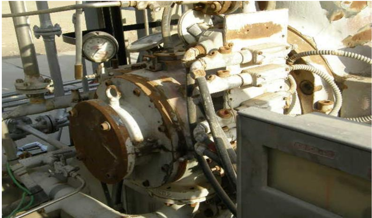
Picture Above: Drive Mechanism Removed at NDE Bearing Housing, Blinded with Flange
