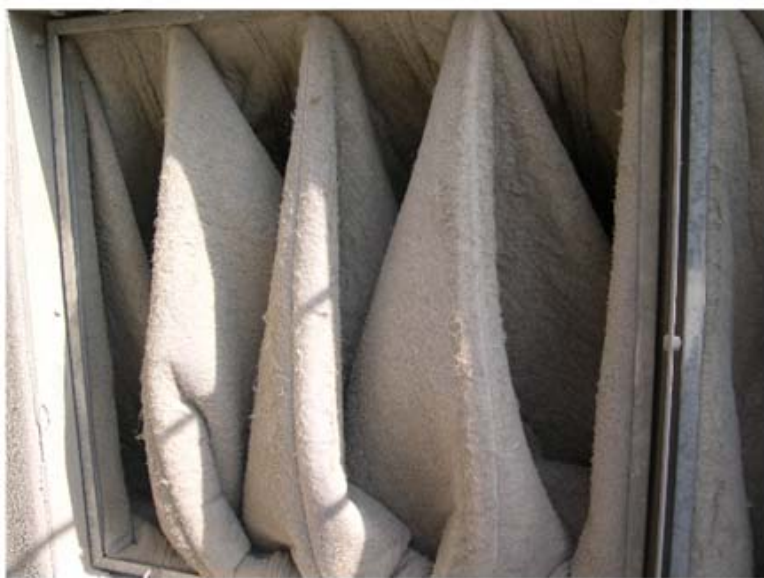
Bag filter loaded with limestone dust
