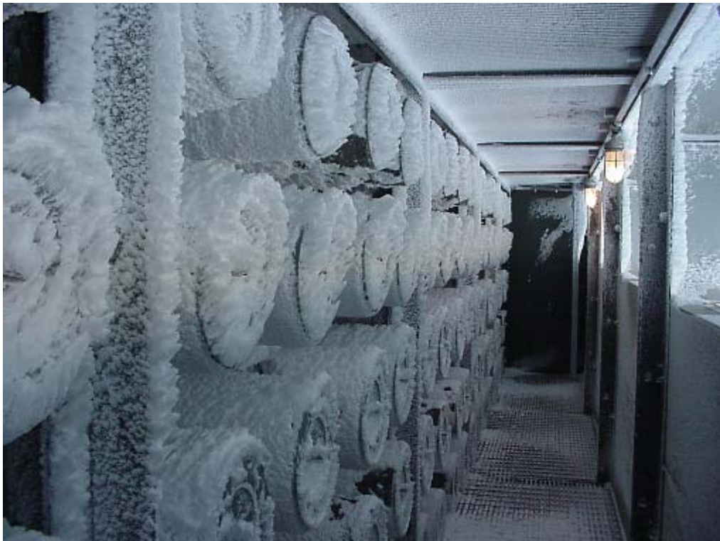
Figure 3-9. Cartridge Filters with Frost Build-Up Due to Cooling Tower Drift (Courtesy of Camfil Farr)
