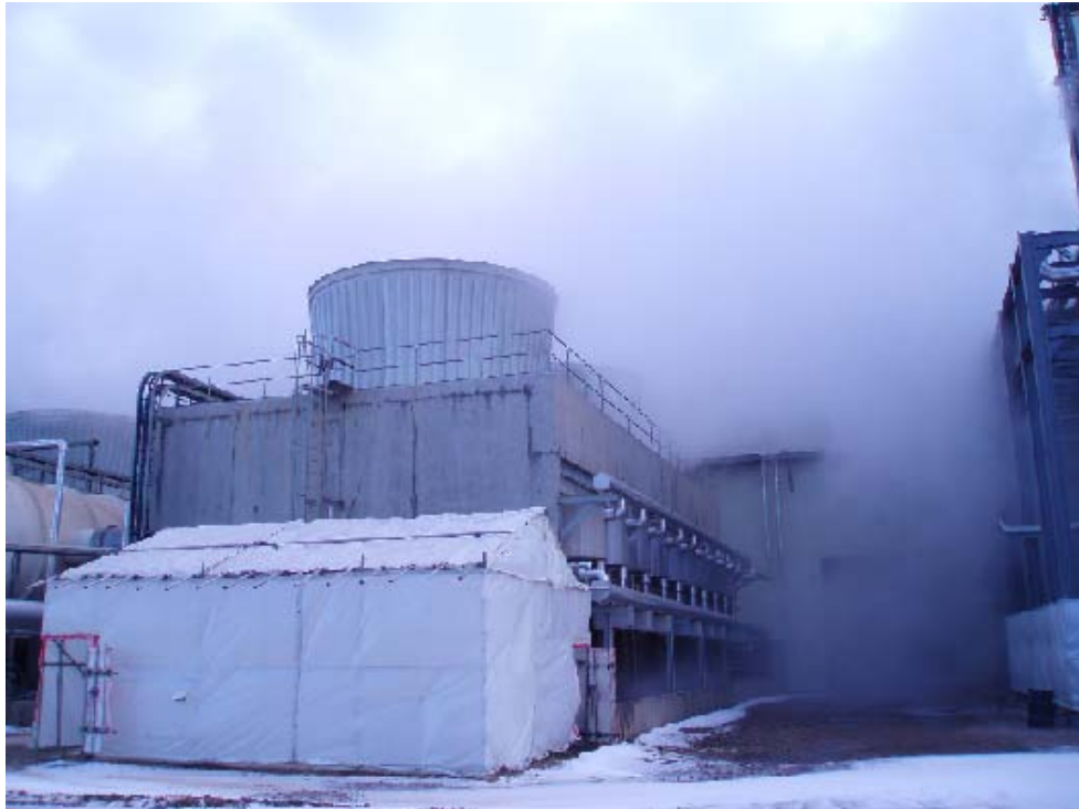
Figure 3-34. Aerosols Drifting from Cooling Tower to Gas Turbine Inlet (Courtesy of Camfil Farr)
